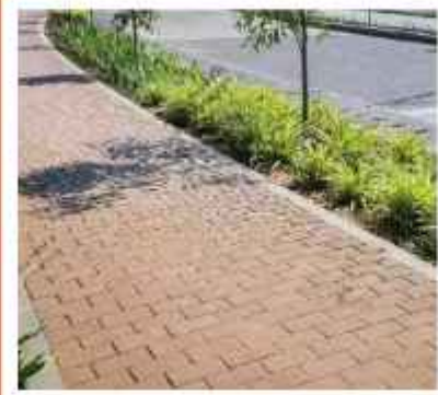
WIDE RCC ROAD BOTH SIDE PAVING
