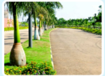
RCC Road with Plantation
