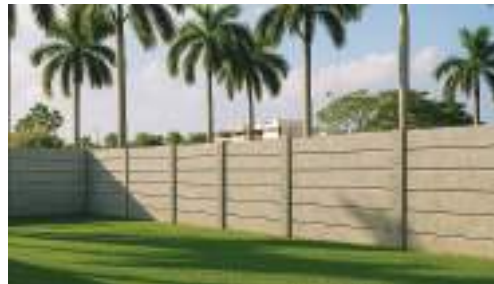
PRECAST COMPOUND WALL
