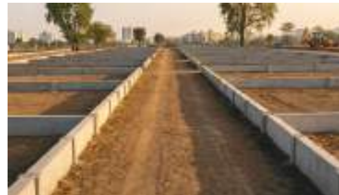
PRECAST DEMARICATION WALL
