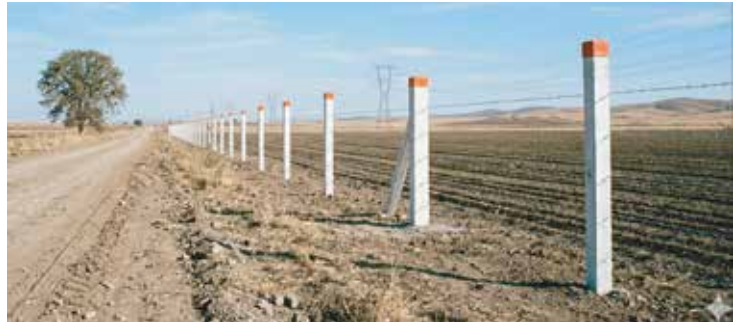
WIRE FENCING WITH POLES AROUND THE PROJECT
