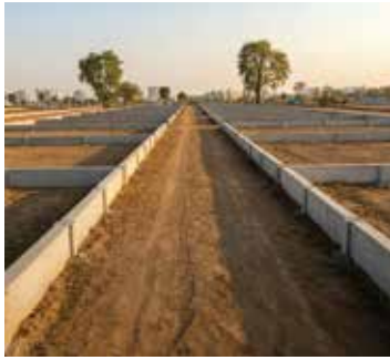
1 FT PRECAST DEMARCATION WALL
