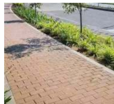
WIDE RCC ROAD BOTH SIDE PAVING
